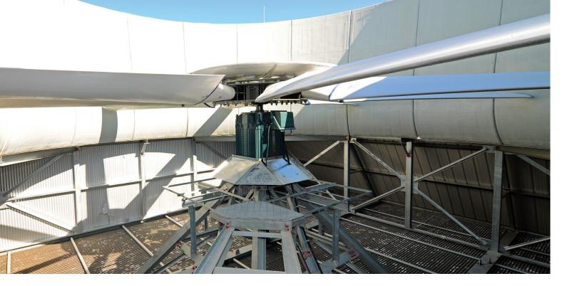
A direct drive motor eliminates many components of a right angle geared system.
