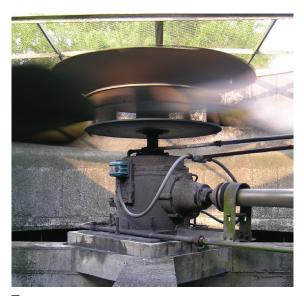
A typical conventional fan drive arrangement of a gearbox mounted under the fan.
